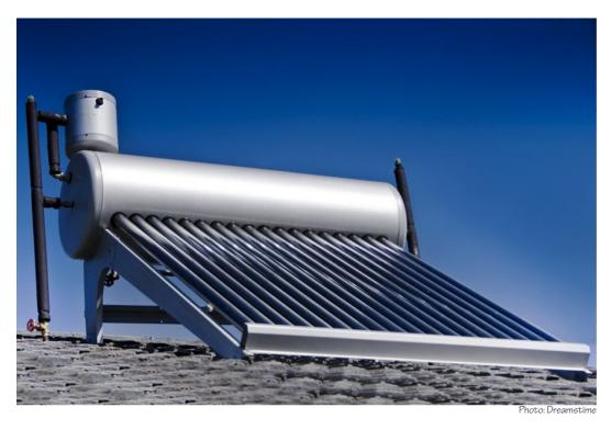
This is a roof-mounted solar water heating unit. These units absorb the Sun's energy to heat water for domestic or farm use. With new and efficient solar hot-water technology, dairy farmers can produce enough hot water to keep all their milking equipment clean, even in the middle of a Canadian winter.
