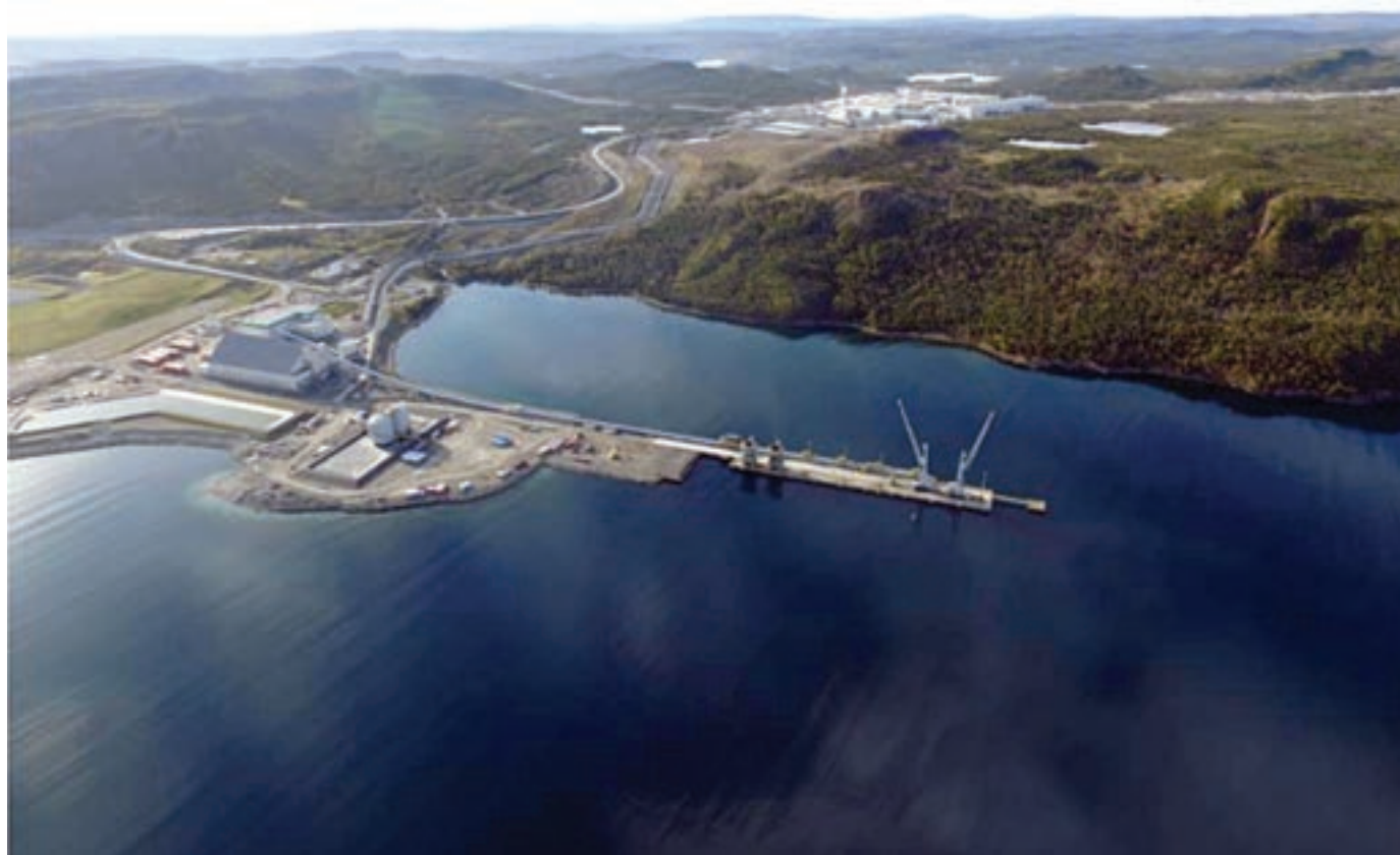
Figure 6: The dock at Long Harbour where concentrate arrives from the Voisey's Bay deposit (Courtesy of Vale).
